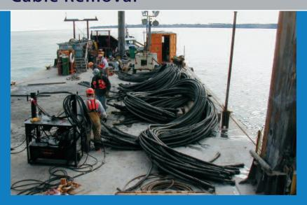
We have removed cable for route clearance, permit requirements, and the removal of out-dated oil-filled cables. The cable materials can be salvaged for scrap, if of value, but will always be disposed of properly in an environmentally acceptable manner.
