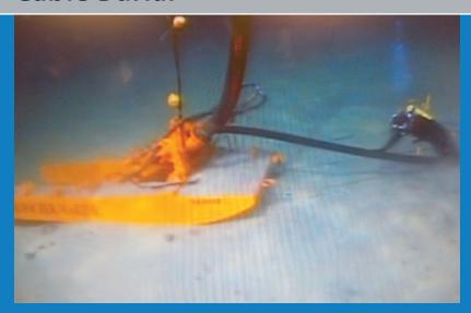
Our jet sleds are capable of burial to 4 meters. These sleds use high pressure water to liquefy the trench for the cable installation. The sleds cause near zero turbidity and are environmentally friendly. They are fitted with the latest underwater technology to continuously monitor the cable burial and installation in real time. These technologies include look ahead sonar, heave, pitch and roll, and GPS tracking sensors.
